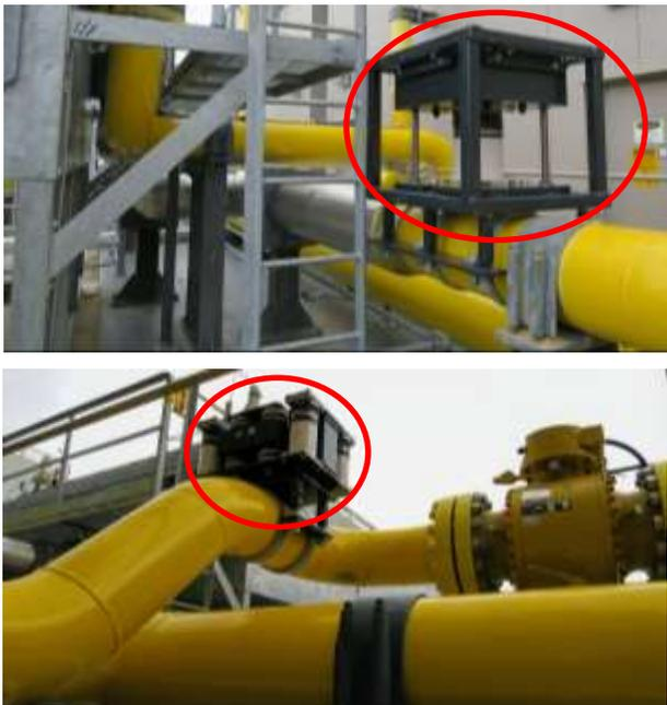
Figure 1 The XY (top) and Z (bottom) TMDs bolted to the pipe
