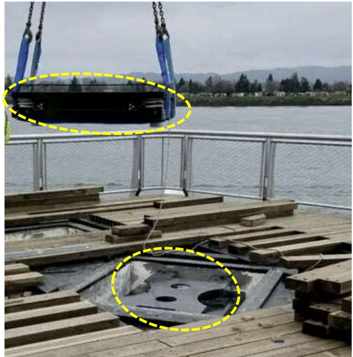
Figure 2 One TMD installed in its cavity and the other one being lowered into its corresponding cavity
