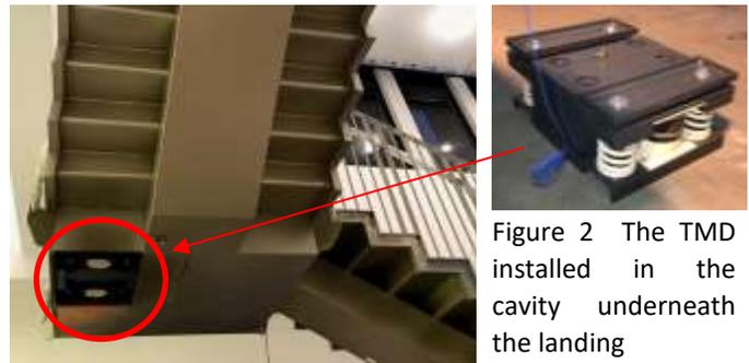
Figure 2 The TMD installed in the cavity underneath the landing
