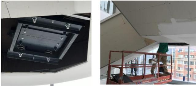
Figure 2 The TMD installed in the cavity underneath the landing (left) and a technician commissioning it (right)
