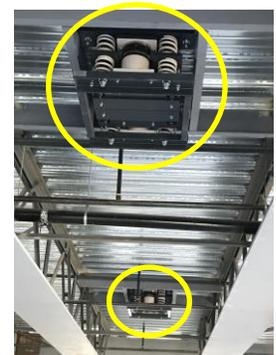
Figure 3 Two TMDs installed underneath one of the bays
