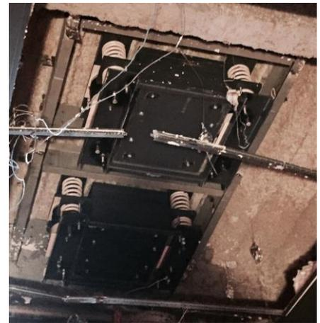
Figure 2 Two TMDs installed underneath one of the bays of the floor system
