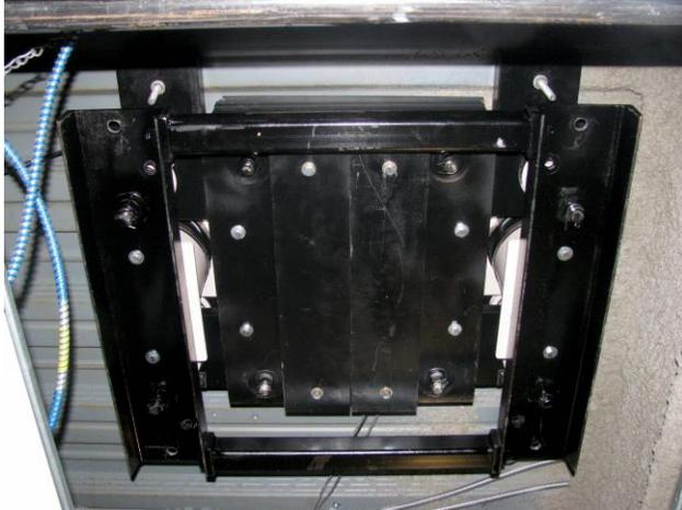
Figure 2 One of the TMDs appended underneath the floor system
