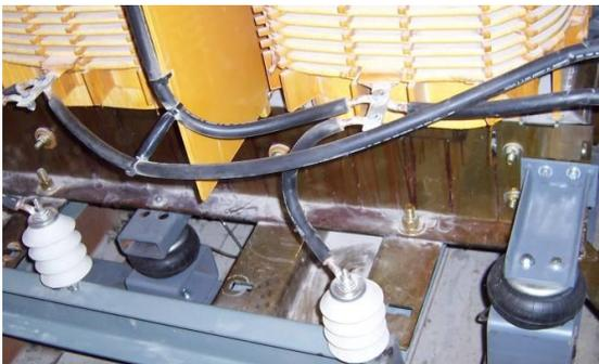
Figure 1 Two of the mounting feet of the transformer
