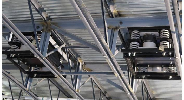
Figure 2 Two TMDs appended underneath one of the floor of one of the classrooms
