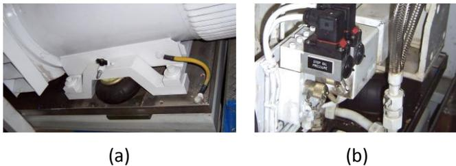
Figure 1. The air mount under the generator (a) and under the diesel engine (b)
