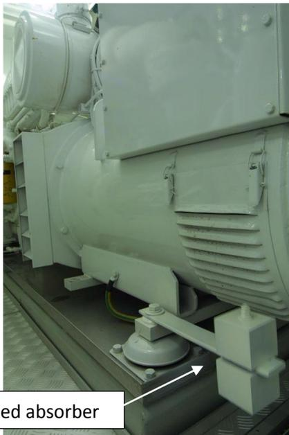
Figure 1 Tuned absorber installed on the front left mounting foot of the diesel-generator
