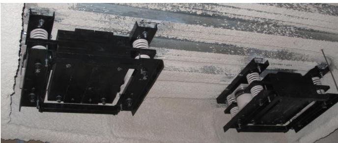
Figure 2 Two TMDs appended underneath one of the balconies
