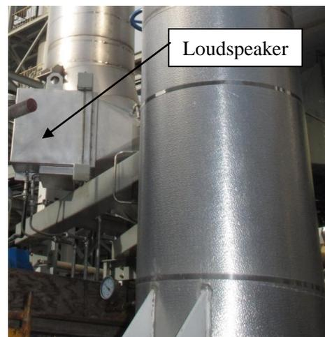
Figure 5 The loudspeaker installed
